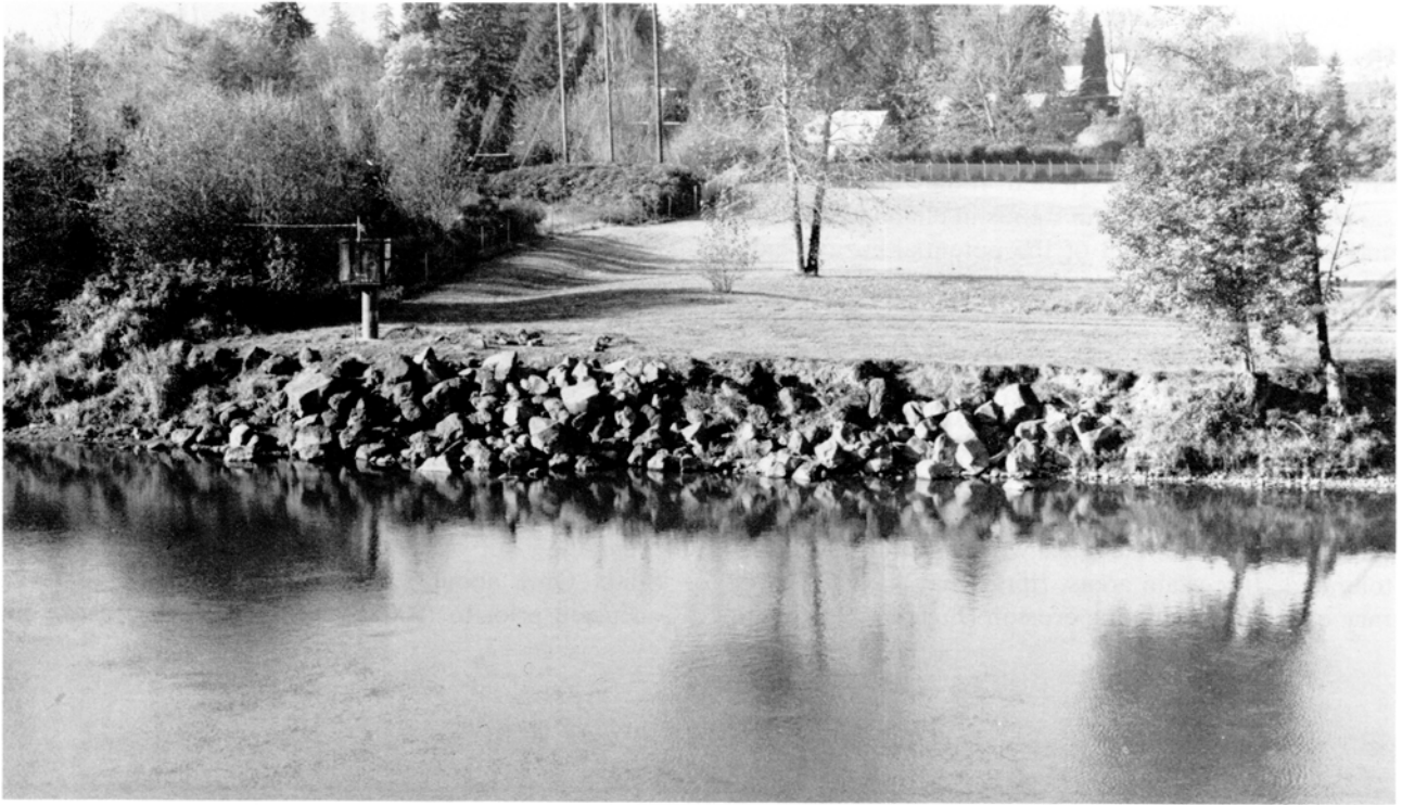
Figure 42. Riprap being used to prevent erosion of north bank of Clackamas River at Clackamet Park.
