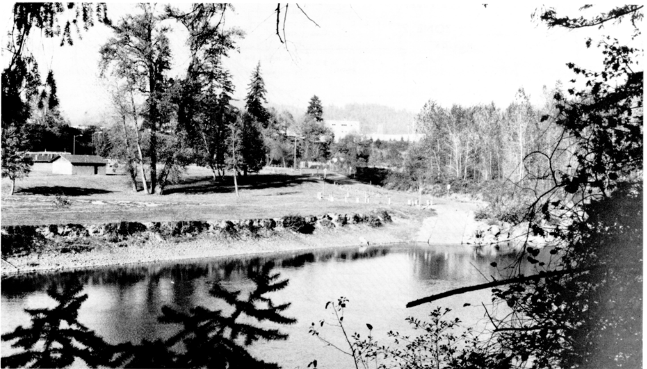
Figure 43. Erosion where banks were not riprapped at Clackamet Park.
