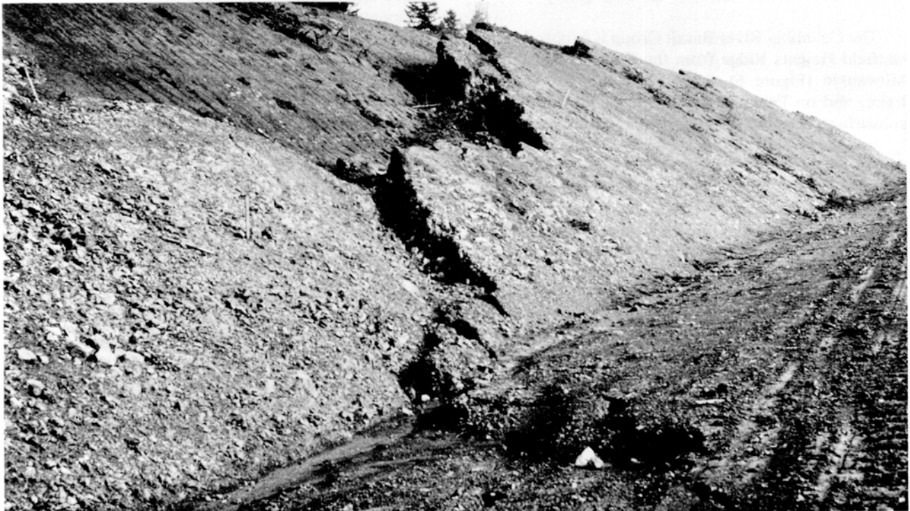
Figure 8. Closeup of same landslide. Weathered Columbia River basalt (Tcr) overlying Vantage horizon failed during construction of large cuts.
