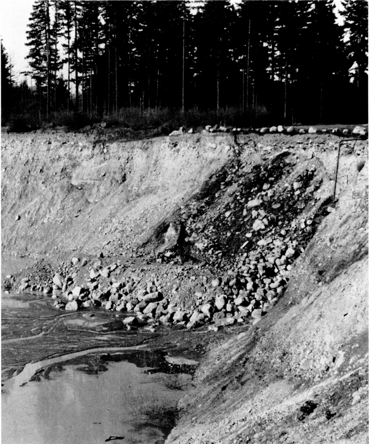
Figure 23. Deltaic gravel (Qdg) in old pit northwest of intersection of I-5 and Carman Road. Photo taken about 1961. Large unsorted boulders scattered throughout deposit were carried from Lake Oswego channel several miles to right (east) of site shown in photo. Note pollution of standing ground water from discharge pipe near upper right margin.
