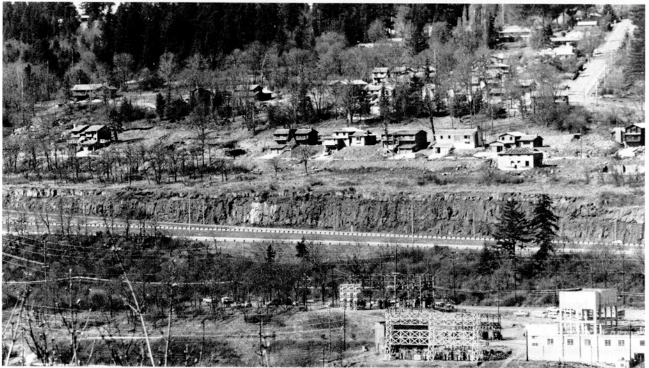
Figure 10. New housing development in West Linn, southwest of I-205 bridge. Freeway cut is in Columbia River basalt (Tcr). Steep cut slopes may present rockfall hazards. Weathered basalt and residual boulders overlie basalt at building site.
