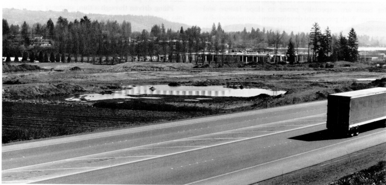
Figure 30. Omark industrial park development area on Minthorn Creek, 1 mi east of Milwaukie. Problems caused by organic soils and high water table have been considered during construction at this location.
