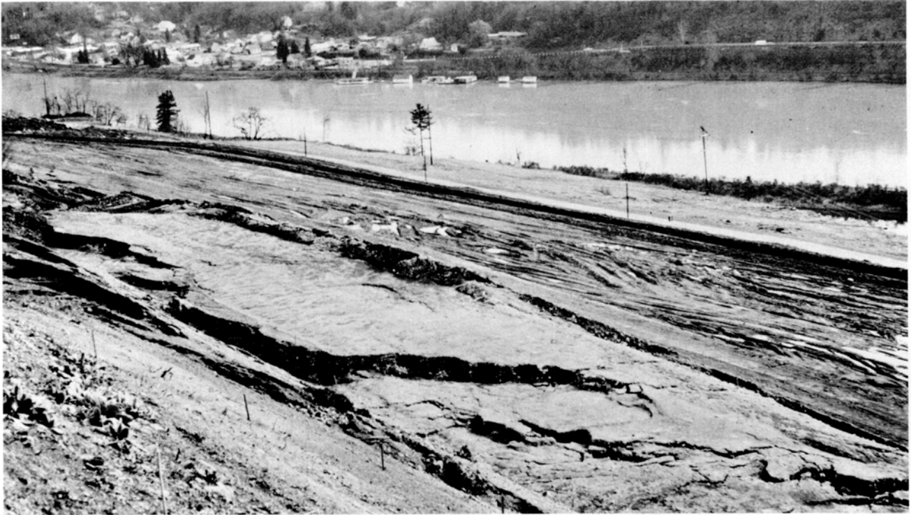
Figure 7. Landslide destroyed cut slopes and roadbed during I-205 construction 1 mi south of Willamette River bridge in West Linn. Several million cubic yards of material had to be removed to correct slide problem.
