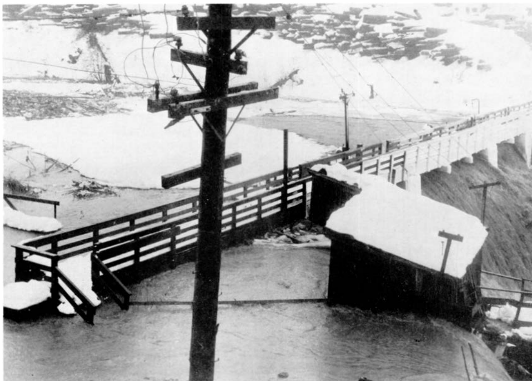
Figure 26. Debris jam at Dee during 1964 flood diverted water through generator station. (Photo courtesy Hood River News )
