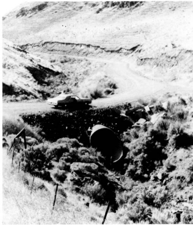
Figure 34. Large culvert used in repair of Fulton Canyon Road after 1964 flood.
