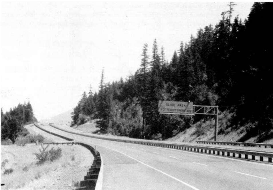
Figure 16. Highway I-80N passes over toe of large slump 3 miles west of Wyeth. Continuing displacement requires periodic maintenance.
