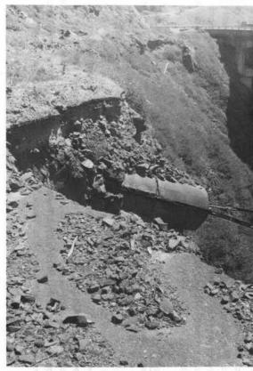
Figure 23. Coastal retreat at Rocky Point has almost totally removed old highway. New highway is bridged over the hazardous terrain at right of photograph.
