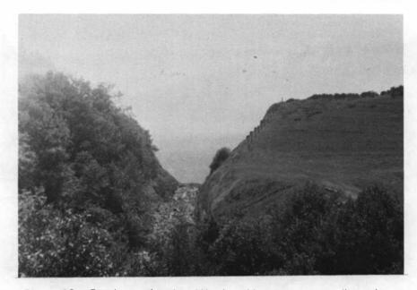
Figure 38. On the south side of Humbug Mountain an overflow channel has been carved out of the slope to direct excessive runoff of Brush Creek directly to the ocean.
