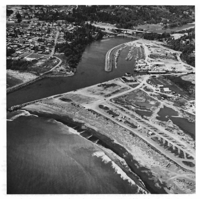
Figure 28. Jetty construction at the mouth of the ChetcoRiver has stabilized the spitand has prompted construction of diverse water-dependent focilities. (Oregon Highway Division Photo)
