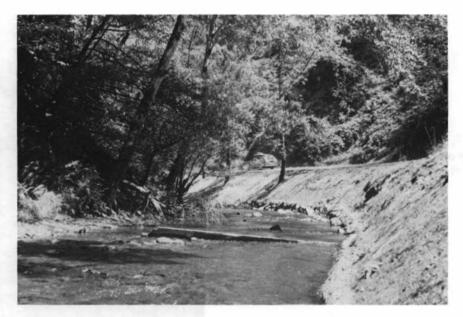
Figure 39. The lower reaches of Brush Creek, downstream from the cutoff channel shown in photo above, are cemented to prevent undercutting of the highway.
