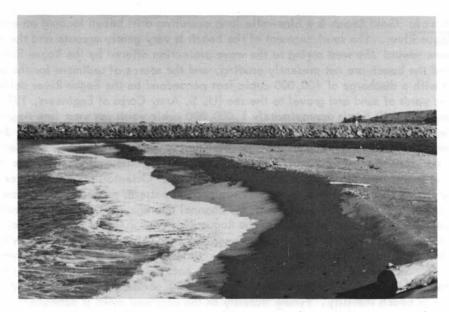
Figure 26. The sand spit and shools between the jetties at the mouth of the Rogue River present severe hazards to navigation.
