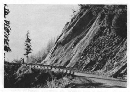
Figure 21. Extremely high rockfall danger on parts of the Rogue River Highway necessitate screening to protect motorists. The hazard is greatest during the winter months.
