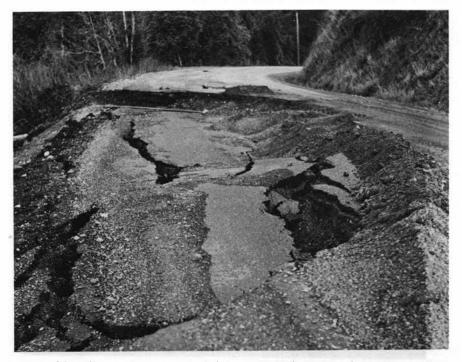
Figure 20. Slumps of road material are commonly caused by stream undercutting, saturation of the fill material, or simply failure of improperly placed fill material.
