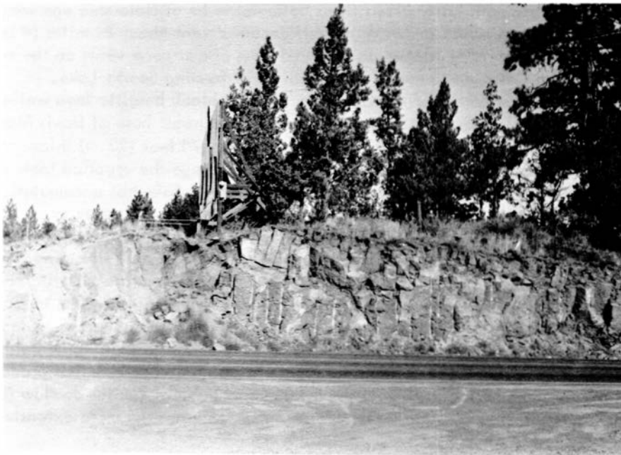
Figure 18. Roadcut north of Bend shows thinness of soil zone and structure of one of the low, rounded tumuli in lavas of the Qb unit and the typical joint pattern in the basalt. Most excavations for streets and utilities in Bend and Redmond encounter this lava.
