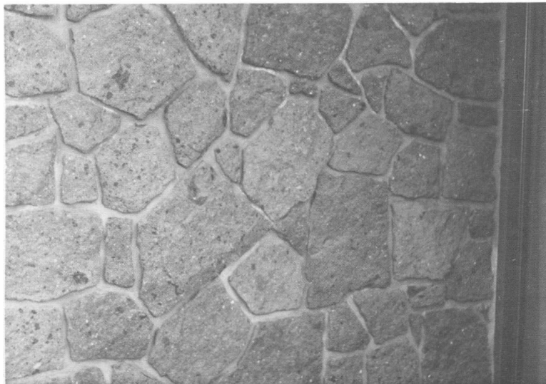
Figure 44. The welded portion of the black ash-flow tuff readily splits into roughly rectangular slabs of rubble stone. Here it has been used as wall veneer for a bank in Bend.
