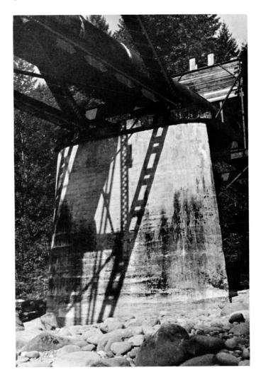
Figure 42. West end of aqueduct crossing downstream from Dodge Park is founded on alluvial gravels.
