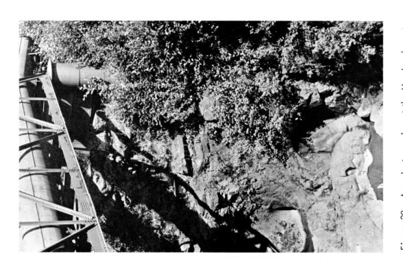
Figure 38. Aqueduct crossing at the Headworks rests on stable Columbia River Basalt.
