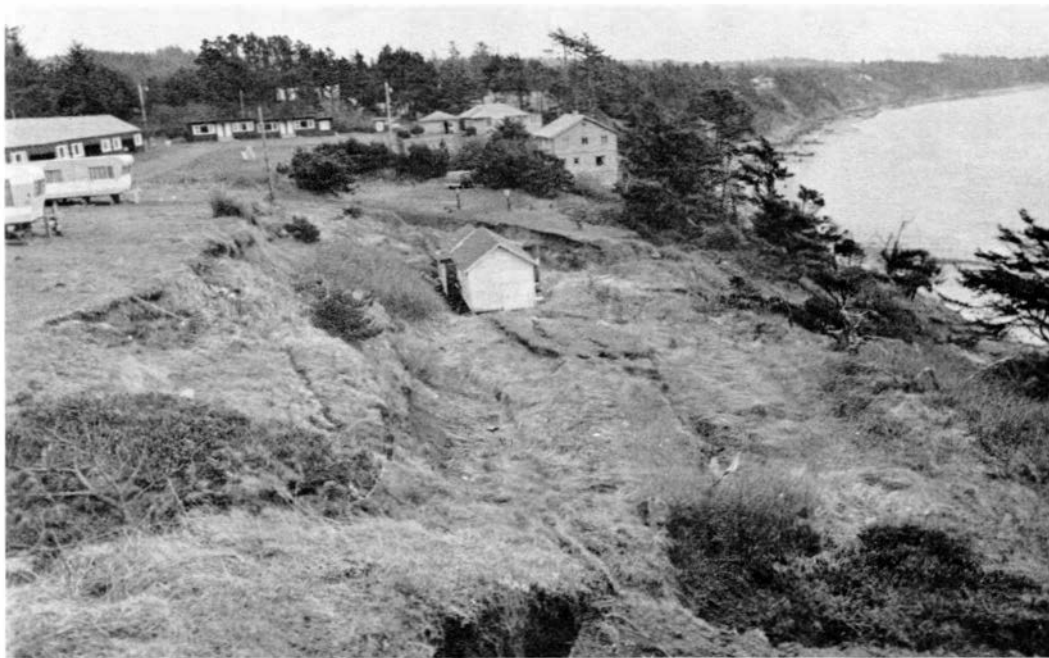
Photo 42. Building in center of photo severely damaged when caught in active landslide at Agate Beach. Ground disruption continues.
