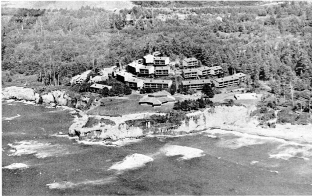
Photo 91. Inn at Otter Crest complex at Cope Foulweather. Upper buildings are situated on basaltic rock. Restaurant is on eroding marine terrace. Erosion is accelerated by landsliding of terrace sediments on seaward dipping sandstone beds.
