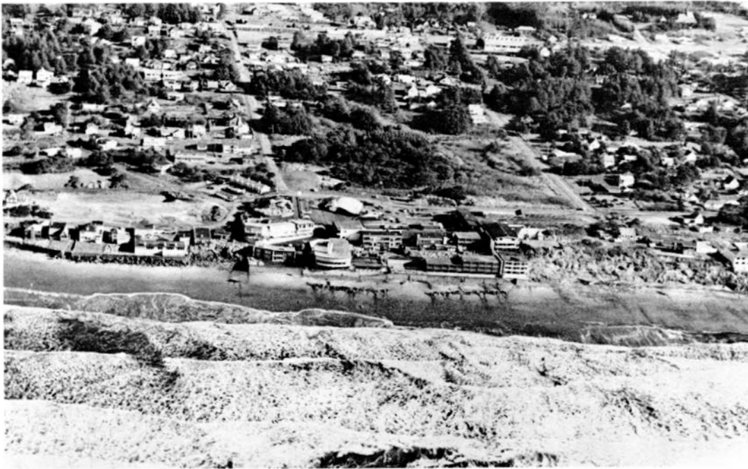
Photo 77. Sea walls and riprap protect some parts of low terrace in Lincoln City. High unprotected terrace to right of photo suffers from extensive wave erosion
