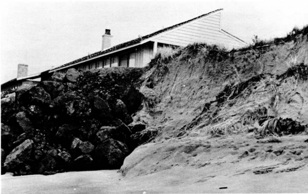
Photo 65. Close-up of house on right side of Photo 63 showing riprap placed to protect property from further storm-wave damage in December 1972.
