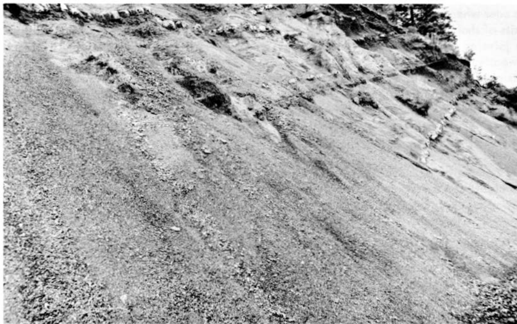
Photo 7. Nye Mudstone on Yoquina Boy road showing characteristic ravelling that produces talus at foot of cuts. Light-colored beds about 1 foot thick are limy concretions.
