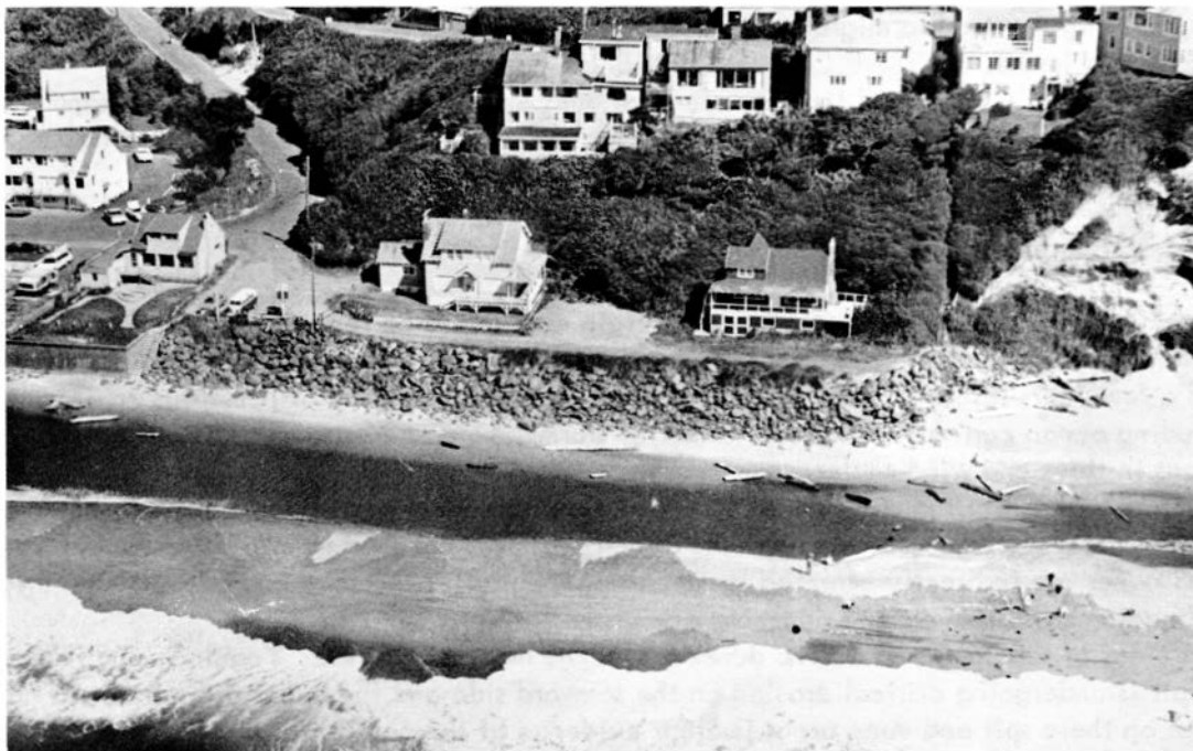
Photo 81. Riprap and concrete sea walls are effective in preventing wave erosion; however, riprap, although less expensive to install, is less resistant and requires periodic repair.
