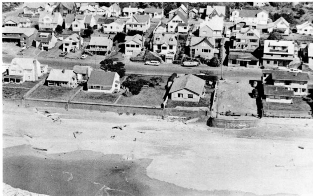
Photo 79. Sea walls in this part of Lincoln City are effective in protecting houses and property on low terrace from wave erosion.
