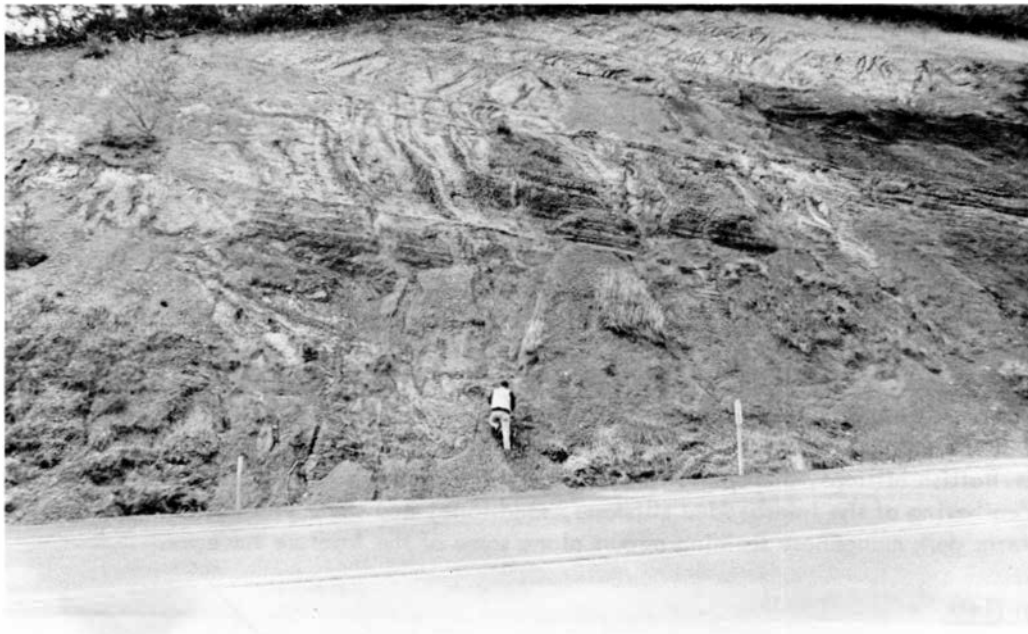
Photo 3. Yamhill Formation exposed in roadcut on Highway 101 near the Lincoln-Tillamook County line. Note characteristic slope ravel in talus deposits at base of cut.
