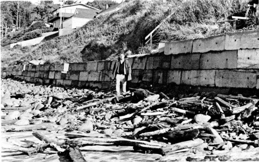
Photo 76. Sea wall at Roods End, consisting of large concrete blocks with weep holes to relieve hydrostatic pressure behind them, provides protection from wave erosion. Sloped bank covered by vegetation prevents sea-cliff recession.
