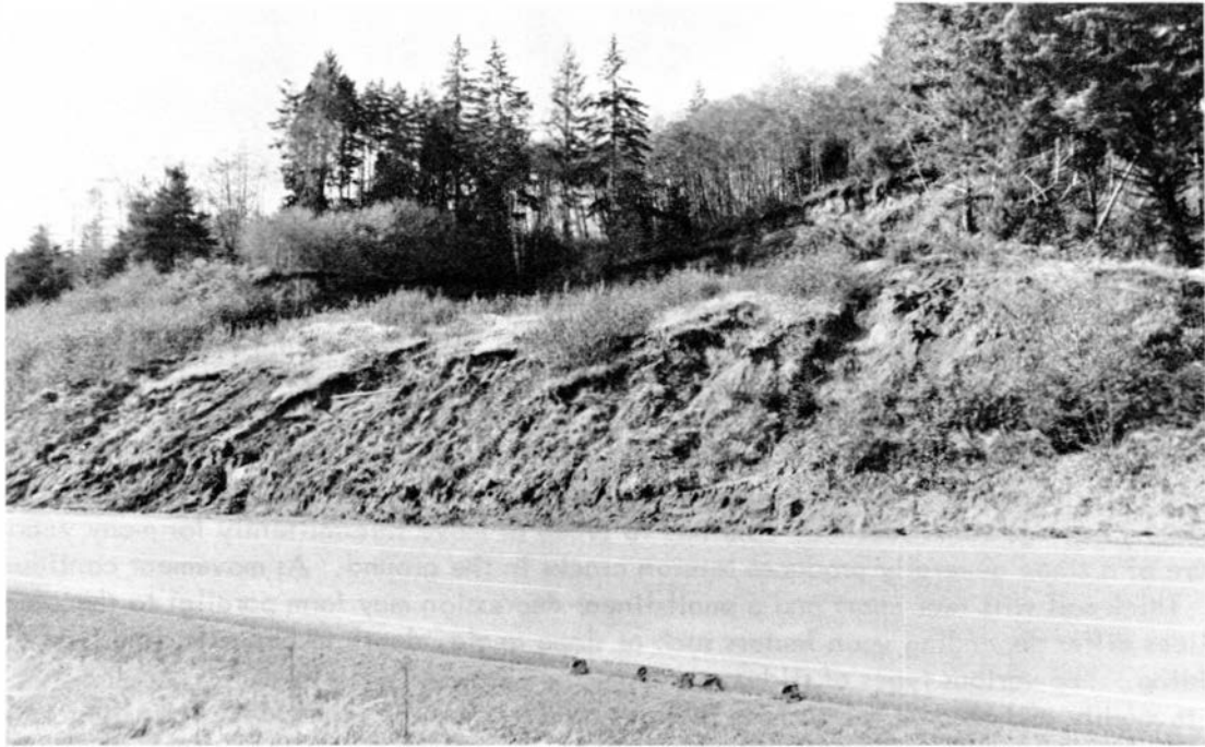
Photo 27. Landslide in roadcut of Highway 101 north of Salmon River. Headscarp of slide can be seen in background. Slide is in residual soils and weathered siltstone of Yamhill Formation.
