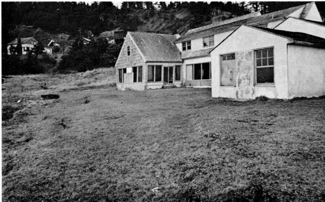
Photo 40. Close-up of house in above photo. Foundation destroyed by break in ground surface visible in right-center of photo. Breaks in ground at left of photo are headscarps of the active landslide.
