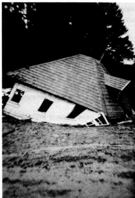
Photo 50. House destroyed when newly constructed highway embankment become saturated and flowed rapidly down a small gully. (Photo by Glen Edenfield, Newport)
