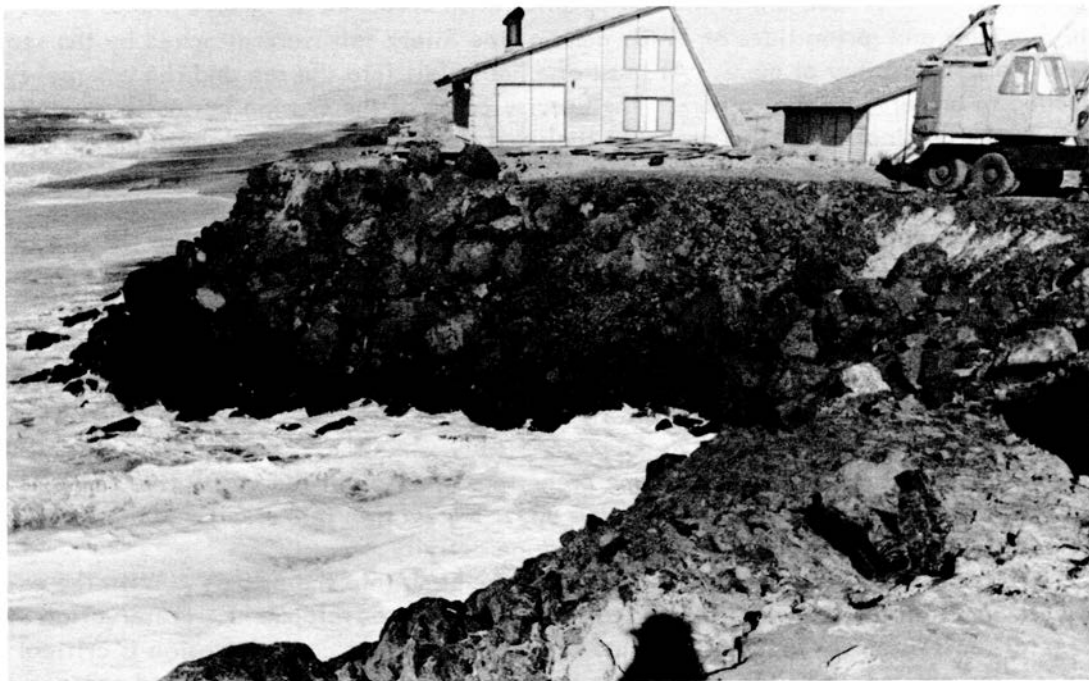
Photo 64. Close-up showing house on left side of above photo where riprap placed earlier at front of house was not sufficient to withstand later storms. Erosion continued to remove sand exposed at either end, requiring additional riprap.
