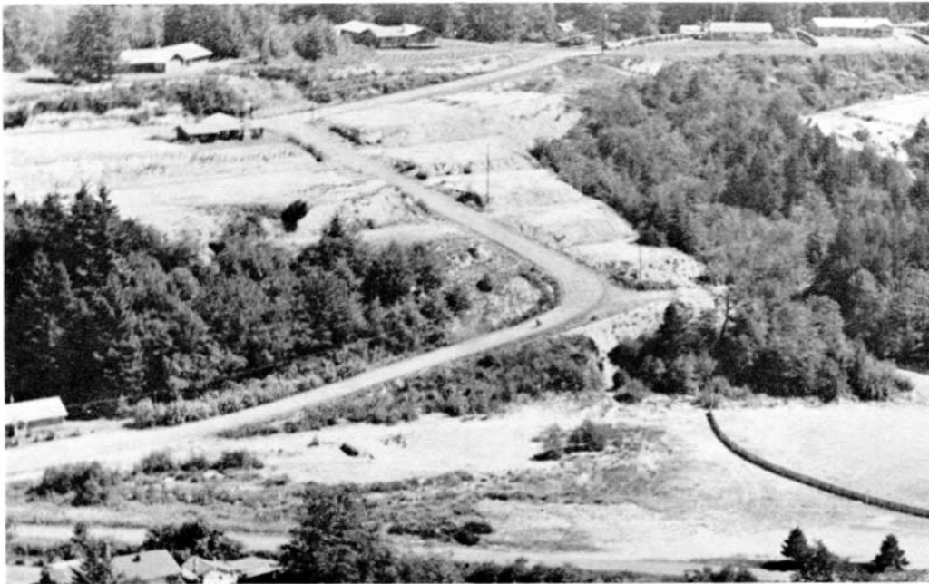
Photo 87. Building pads stairstepped on hillside in Waldport. Such development will require control of surface drainage to prevent erosion and landsliding. Embankments must be properly compacted and have adequate subsurface drainage.
