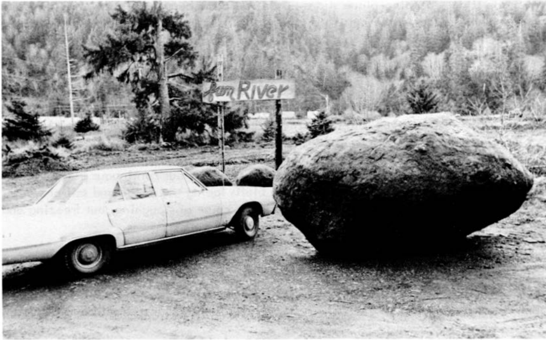
Photo 29. Large boulder from Siletz River Volcanics loosened during winter rains of 1973 rolled onto Siletz River Road at Fun River.
