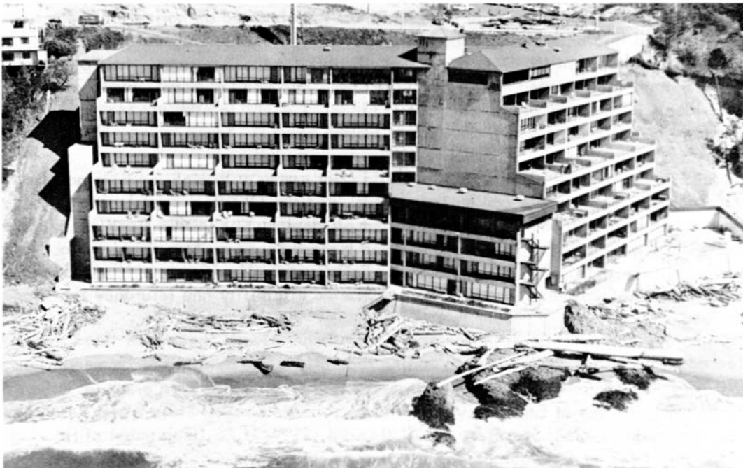
Photo 92. Inn at Spanish Head condominium near Taft. The lower floor is highly vulnerable to the force of storm waves and driven logs.
