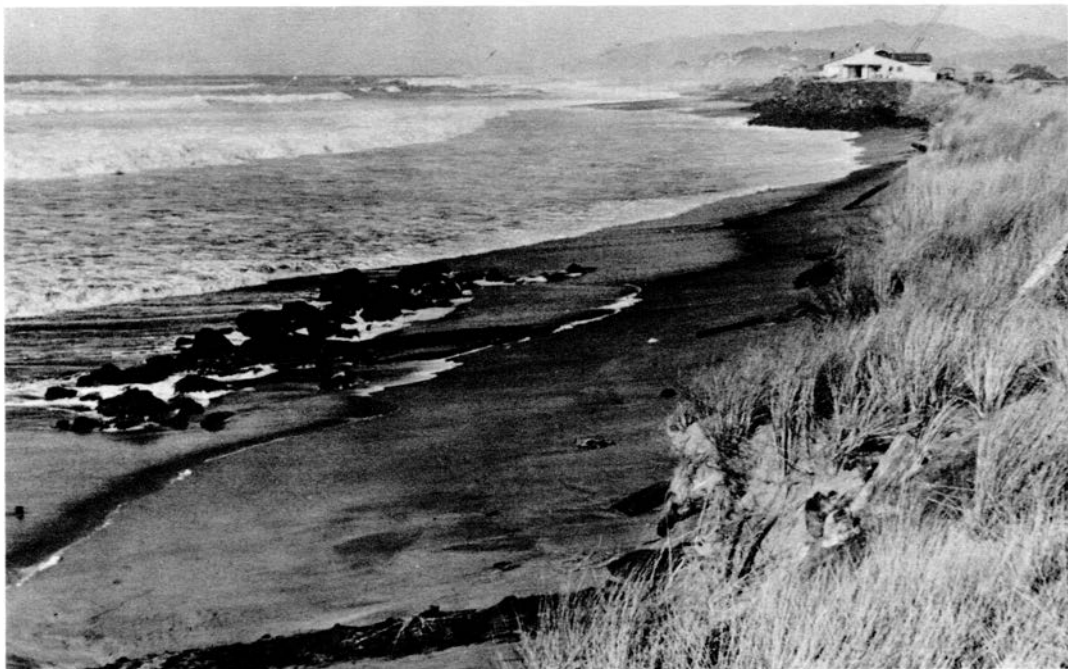
Photo 72. Even riprap placed along a lot frontage failed to prevent wave erosion of dune sand. Evidently at this site erosion worked behind riprap boulders.
