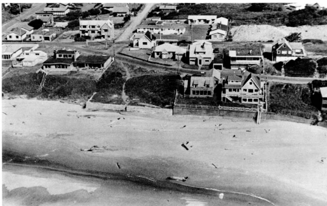
Photo 78. Sea walls stabilize some sections of Lincoln City's coastal terraces, while other sections are exposed to wave erosion.
