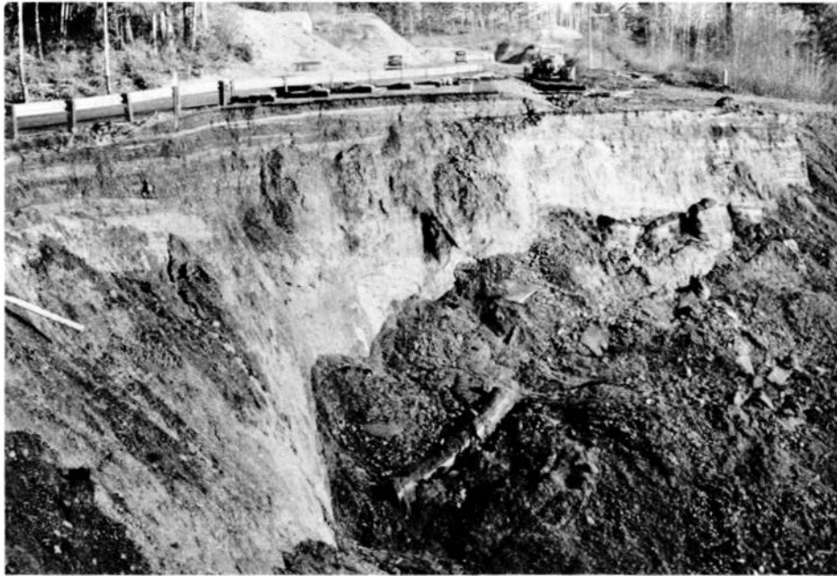
Photo 49. Embankment failure in recently constructed highway 1 mile east of Newport caused by impaired drainage of Nye Mudstone at base of fill.
