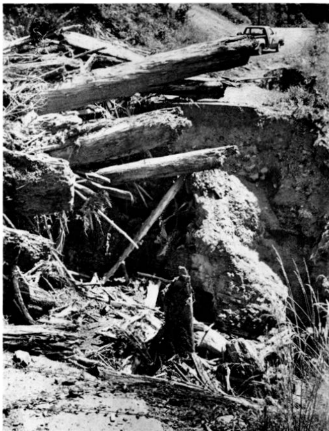
Figure 39. Washout of the Trask River Highway (sec. 6, T. 2 S., R. 7 W.) caused by the winter storms of 1972. High flow of the Trask River (right of photo) was not a factor. All damage was caused by flash flooding of a small, seemingly insignificant side channel.
