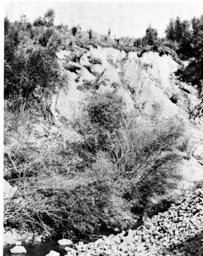
Figure 29. Riprap in foreground acts to protect the road (not shown) from stream erosion, but it also directs stream flow against the toe of the slide. The degree to which this may induce future sliding on the far bank is unknown.
