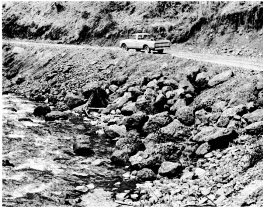
Figure 32. Intense flood activity attacks the stream bank at every turn along Big Creek; here riprap has been placed to protect the road.
