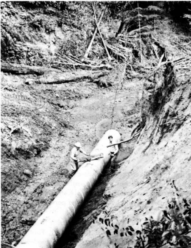
Figure 35. Another view of the same washout. From the extent of the damage to the road and along the creek downstream, it is evident that the new culvert will be insufficient to handle the volumes of water that can be expected in future flash floods.
