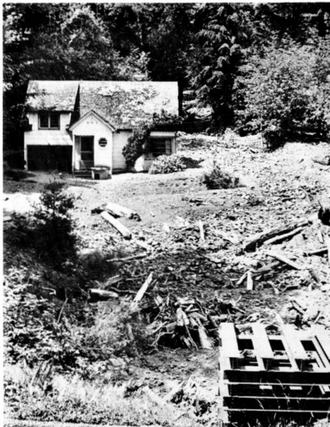
Figure 33. Damaged house partially buried in debris brought down Negro Jack Creek (sec. 8, T. 1 S., R. 8 W.) during the floods of 1972. Conditions along the creek conducive to flash flooding include short channel length, steep slopes, and impermeable bedrock.
