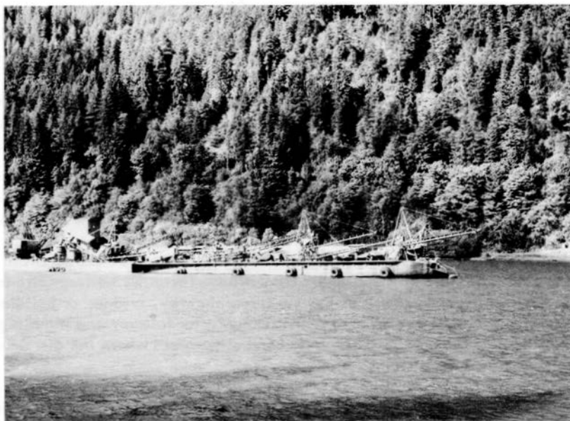
Figure 19. Umpqua River Navigation Co. dredging operation on the Umpqua River near mouth of Indian Charlie Creek about 10 miles east of Reedsport. Equipment includes clam-shell dragline, barge-mounted screening plant, and conveyor belt for loading barges.
