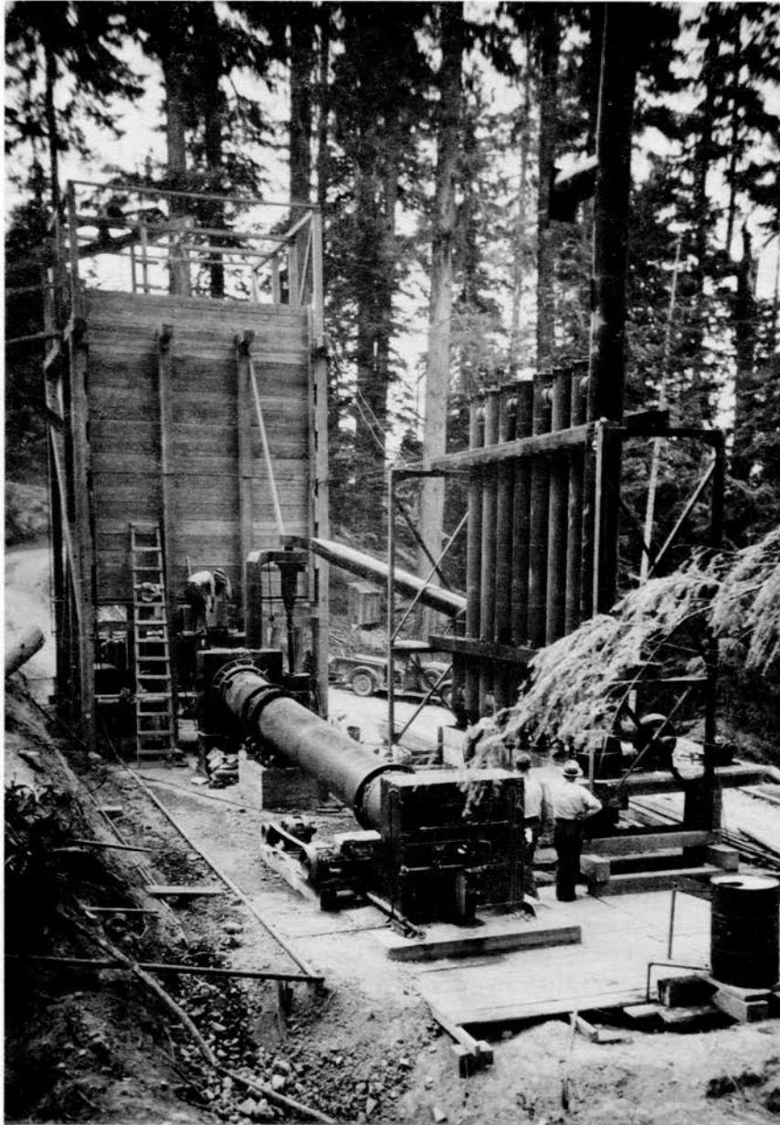
Figure 10. Rotary furnace at the Red Cloud mine about 1940.
