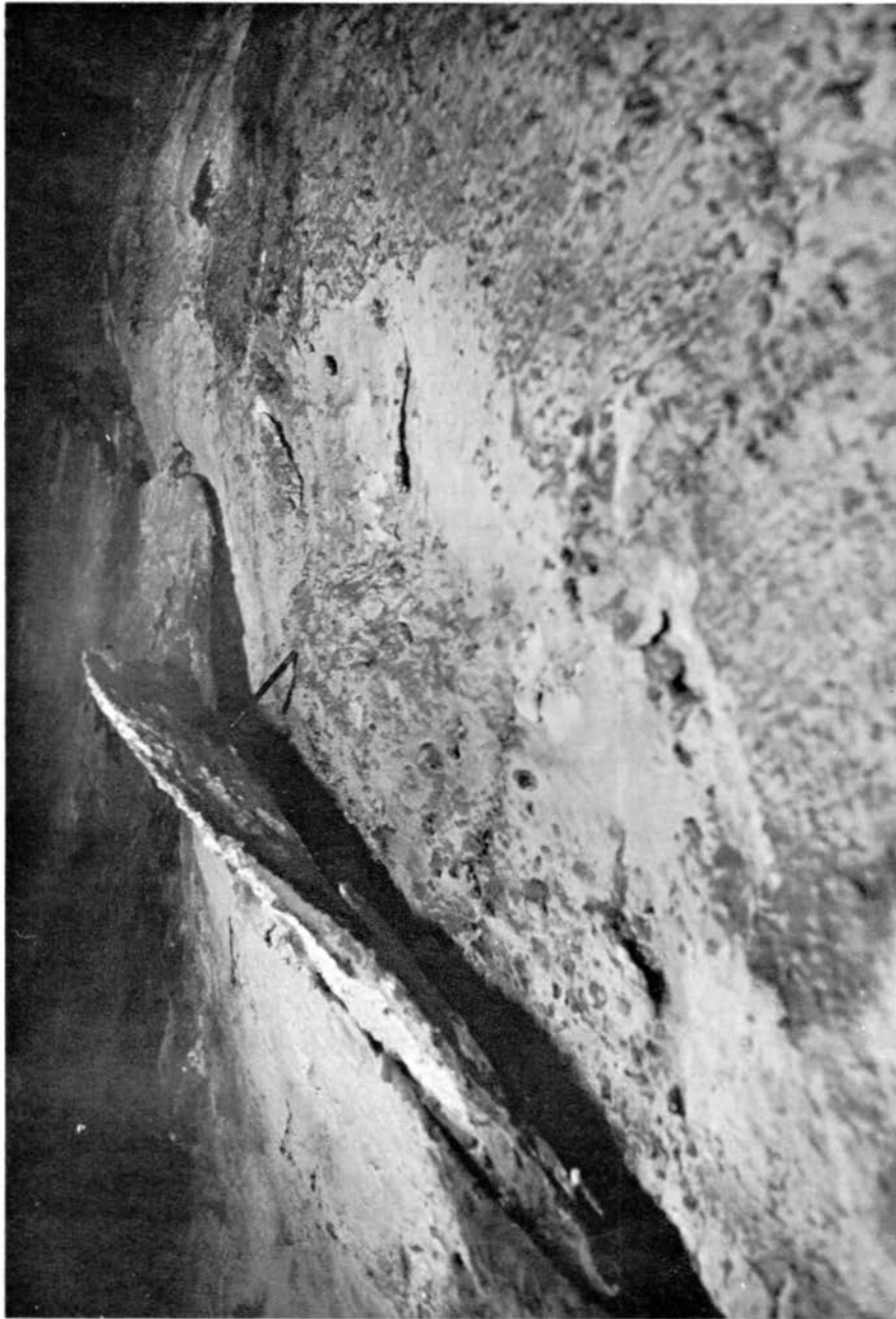
Figure 15. Wind Cove, Station 33. Plastic deformation of port of wall lining. Pencil is 13 cm long.
