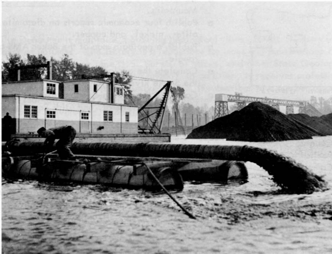
Suction dredging for sand and gravel, Willamette River near Ross Id.
