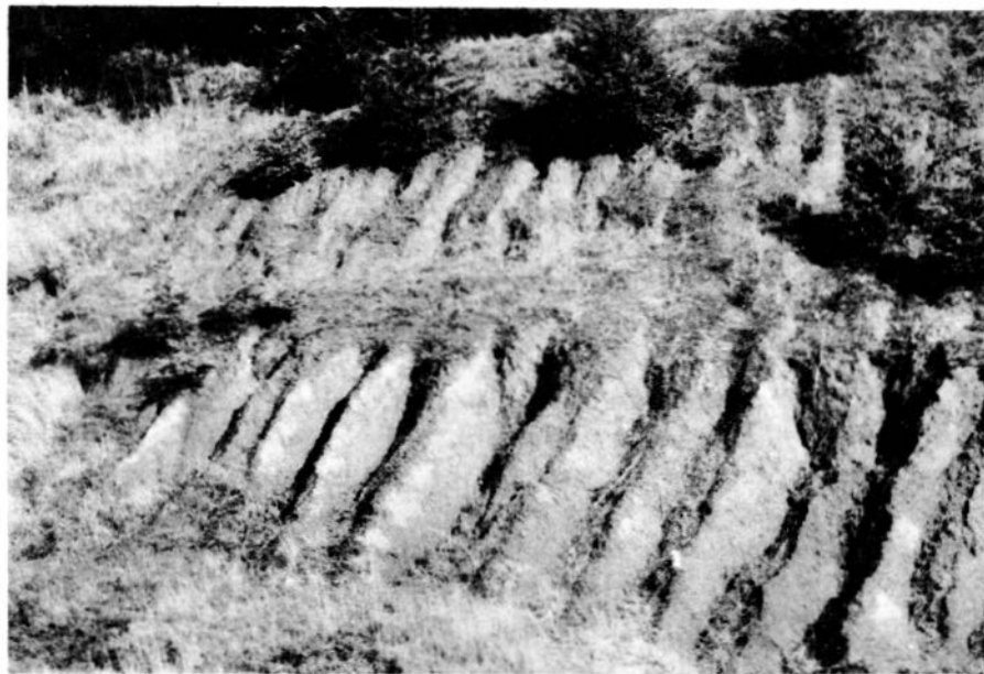
Figure 30. Severe gullying in Helvetia Formation occurs where cut at 1 to 1\frac{1}{2} slope.
