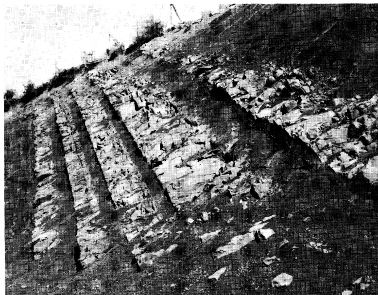
Figure 28. Graded volcanic graywacke beds (upright) and black mudstone of Lonesome Formation in roadcut on Antelope Creek.
