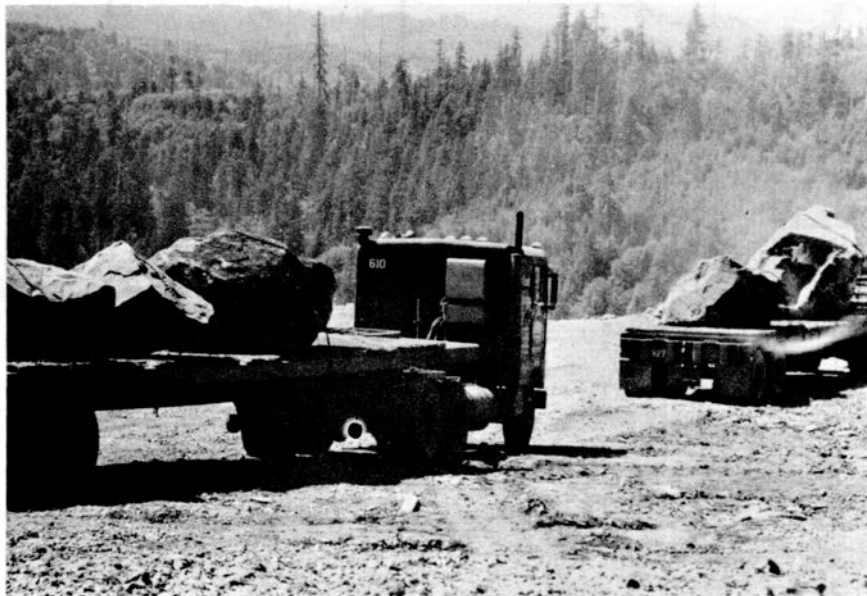
Suitable jetty stone is not easy to find. These huge blocks are from a quarry on the Siletz River, Lincoln County.
