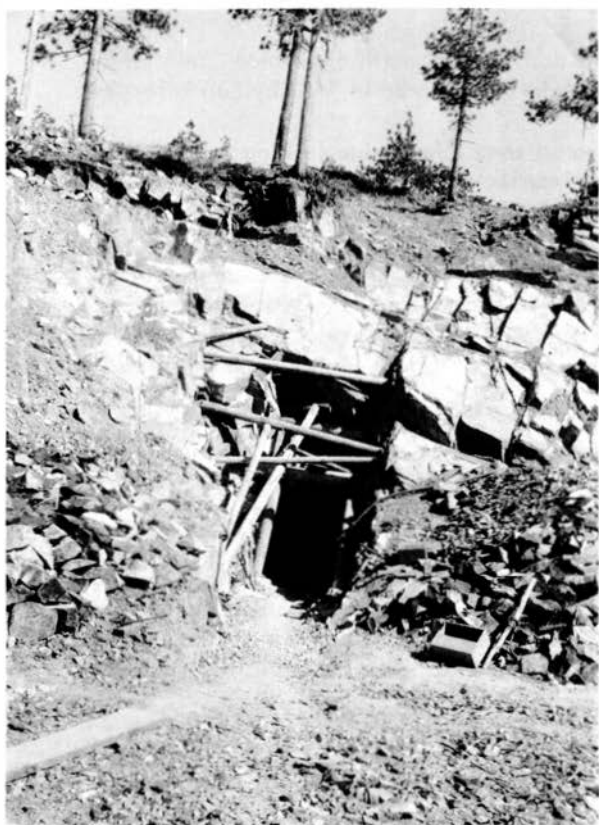
Figure 19. Portal of tunnel in open cut at Lucky L. & R. mine. Note prominent joints in blocky peridotite.
