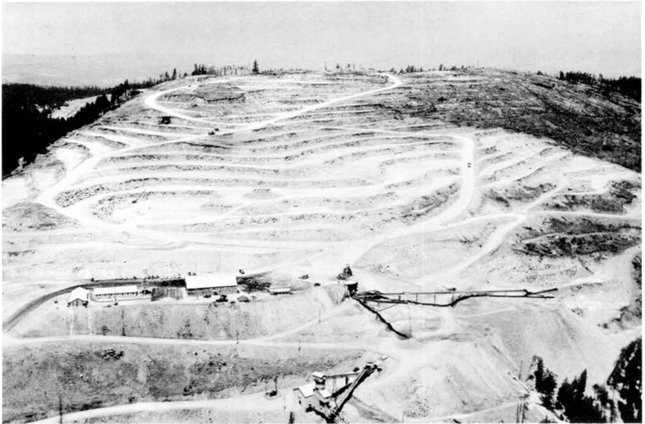
Aerial view of Hanna Mining Company nickel mine, near Riddle, Douglas County, showing open pit benches and aerial tramway leading to smelter.
