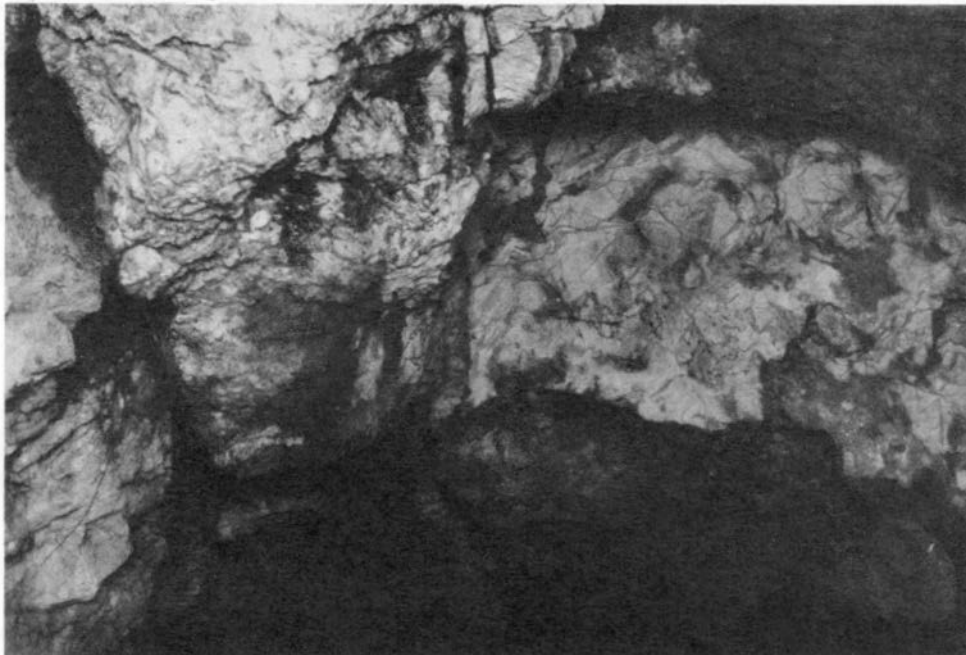
Figure 18 - Cougar mine. Cougar vein, No. 1 tunnel, about 50 feet from portal, looking northward at back of drift. The vein, which is shown on left side of photograph, dips 80° east. On the right side of photograph, a vertical dike is shown coming into the drift from the east wall and then narrowing and turning to follow the vein northward.
