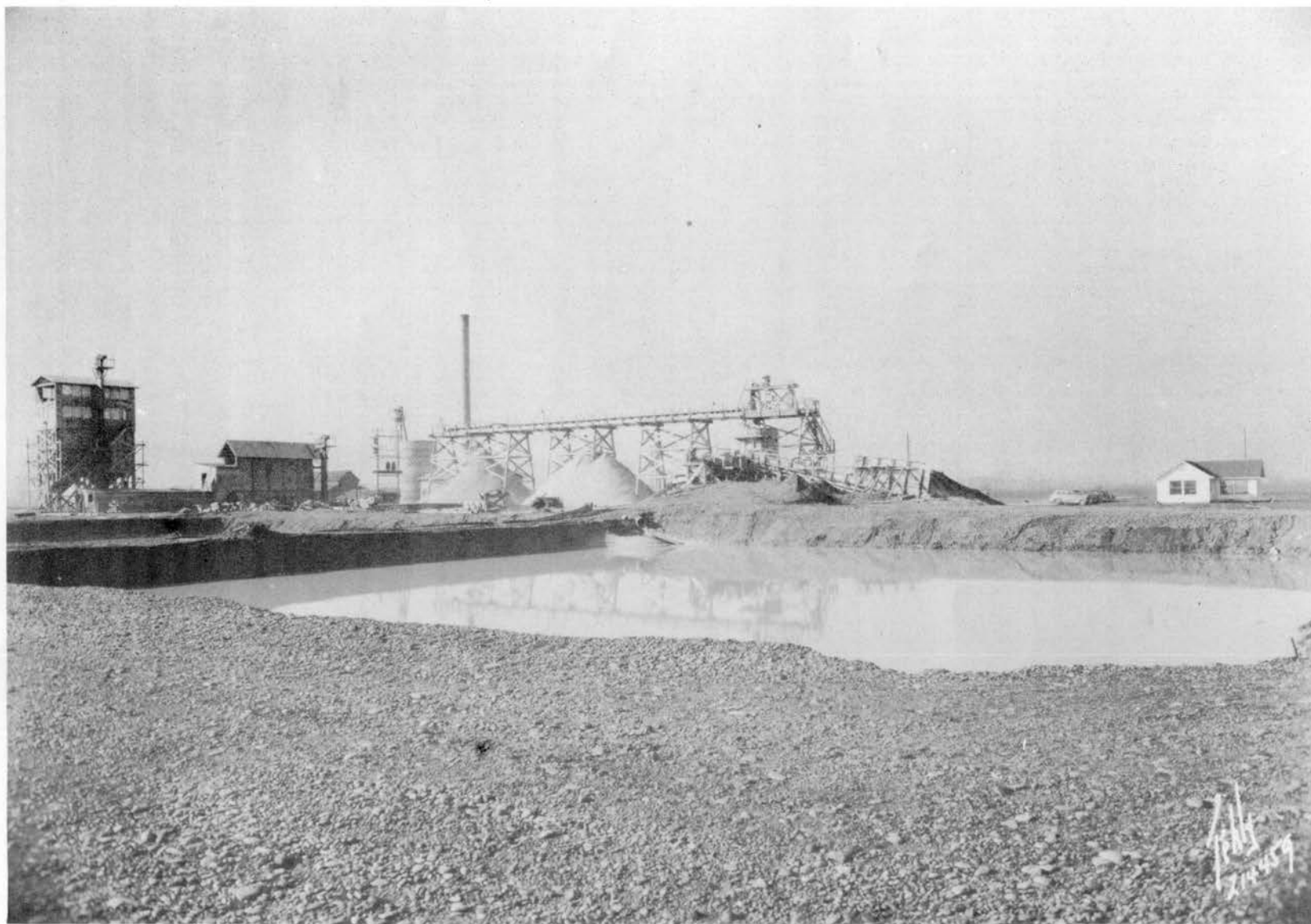
Silica sand washing plant of Silica Products, Oreg., Ltd., Eugene, Oregon, where steel foundry sand is produced.
