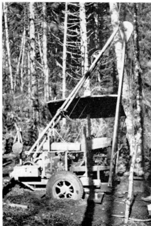
D. Power drill at Englewood project.
