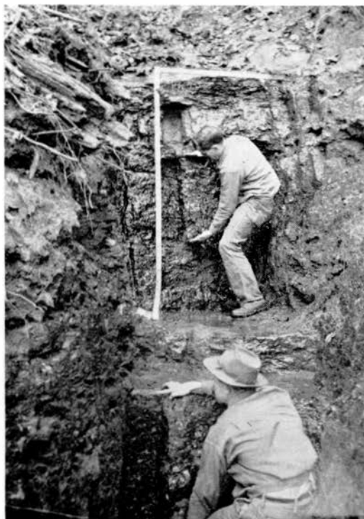
B. Three benches of coal in Cut No. 56. Englewood project (note sampling channels).
