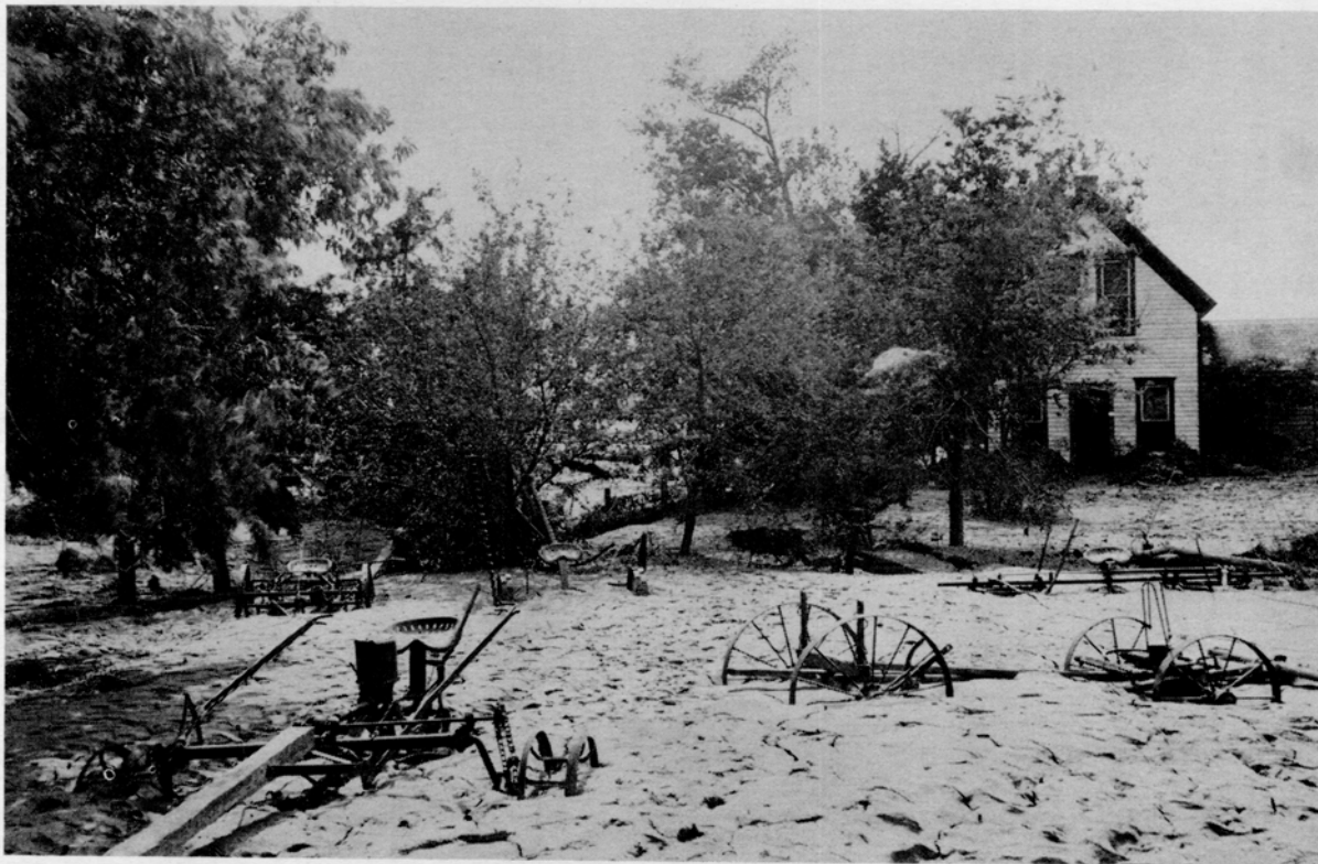
Fig. 12. Deposits made by a single flood over a farmstead on the south bank of the Republican River near Guide Rock, Nebraska. The thickness of the deposits may be judged by the extent of burial of the farm machinery and the deposits which had to be cleared away from the door of the house. This deposition arises from lack of erosion control of the hill lands. (Photograph by the U. S. Soil Conservation Service.)
