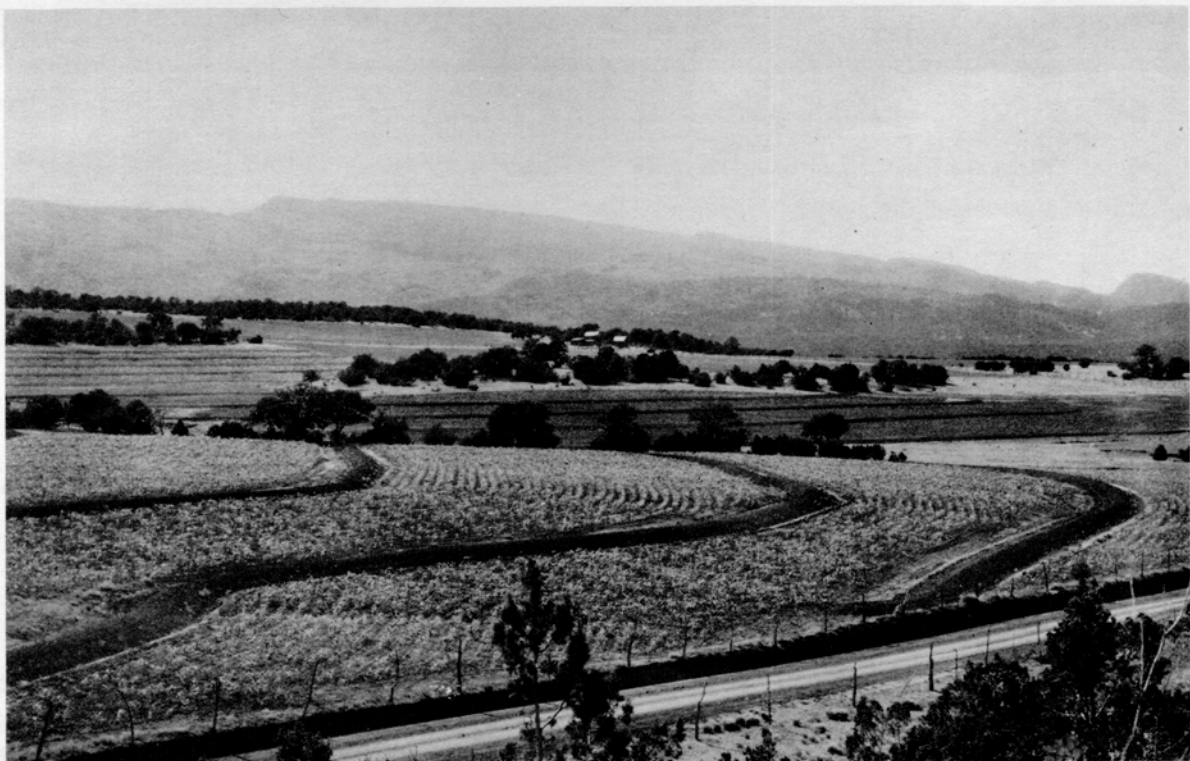
Fig. 24. Terraced land in New Mexico. It should be noticed that the terraces are on the contours, or nearly so. The water is led to the draw indicated by the line of trees. ( Photograph by the U. S. Soil Conservation Service. )
