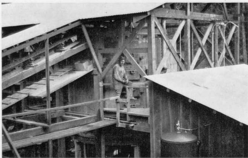
Photo No. 25—The feed belt carrying ore to drying hearth of Bonanza Furnace.
