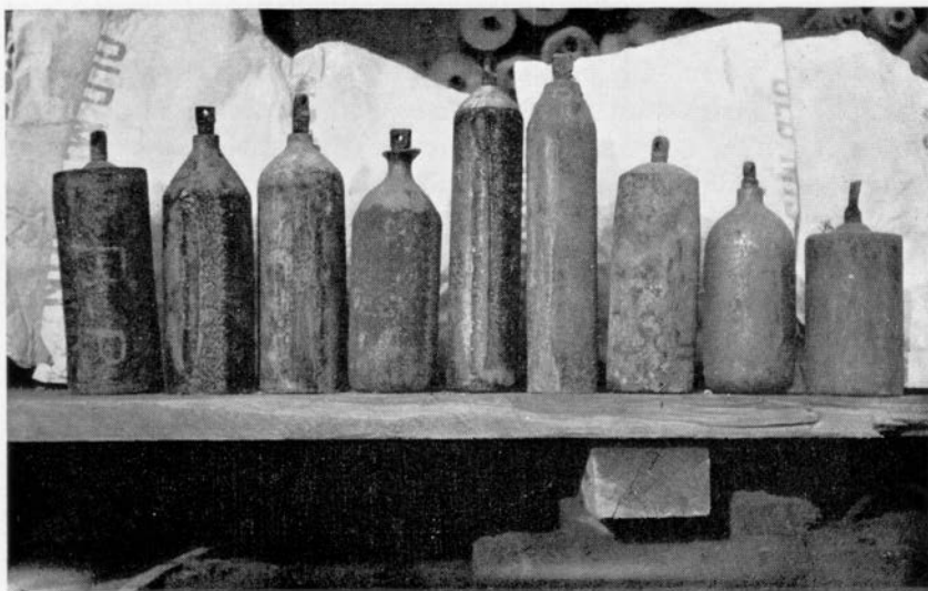
Photo No. 7—Different sizes and shapes of flasks that are in common use. A filled flask holds 76 pounds net, of quicksilver
