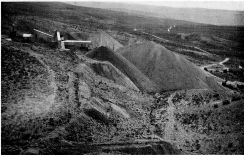
Photo No. 38—The tremendous dumps of burned-rock that have been built up around the Opalite Plant in 11 years of operation. The mine dump of No. 1 Tunnel shows in the foreground.
