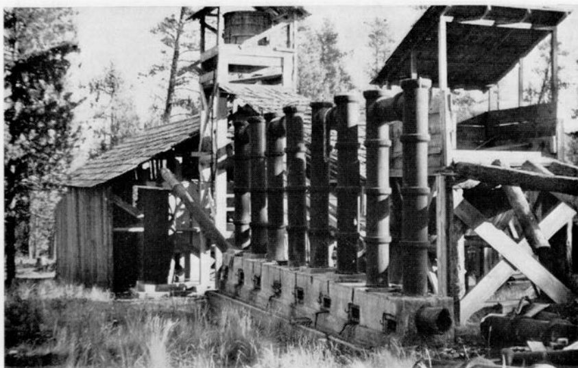
Photo No. 13—This shows the Condenser System of the Rotary Furnace shown in Photo No. 12. It was way too small for the size of the furnace.
