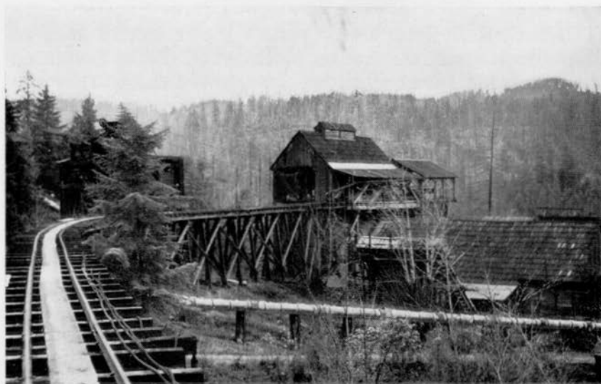
Photo No. 35—General View of the Black Butte Plant. It shows the railroad from the Dennis Creek Tunnel, the aerial tram, new stack at left, old stack flue in foreground, and condensers at the right.
