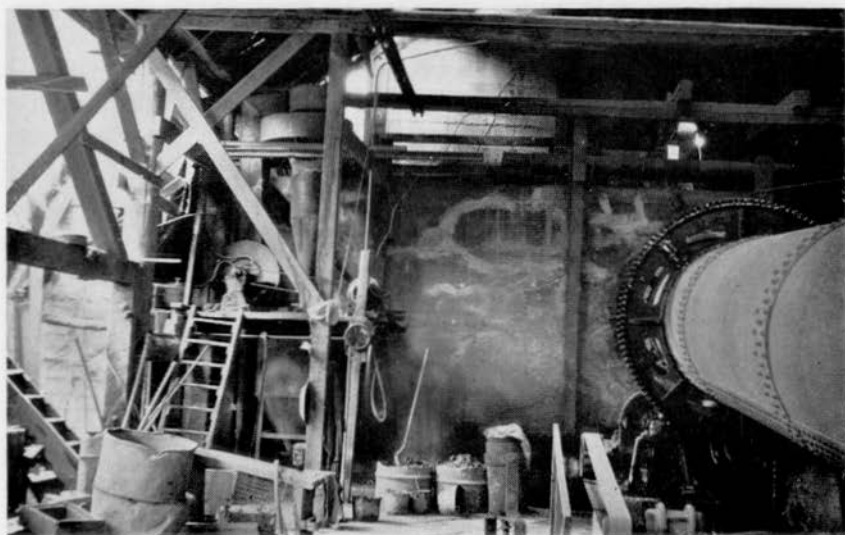
Photo No. 34—The original rotary kiln at the Black Butte Plant. Note the newly added "Sirocco" dust collector at the upper left.
