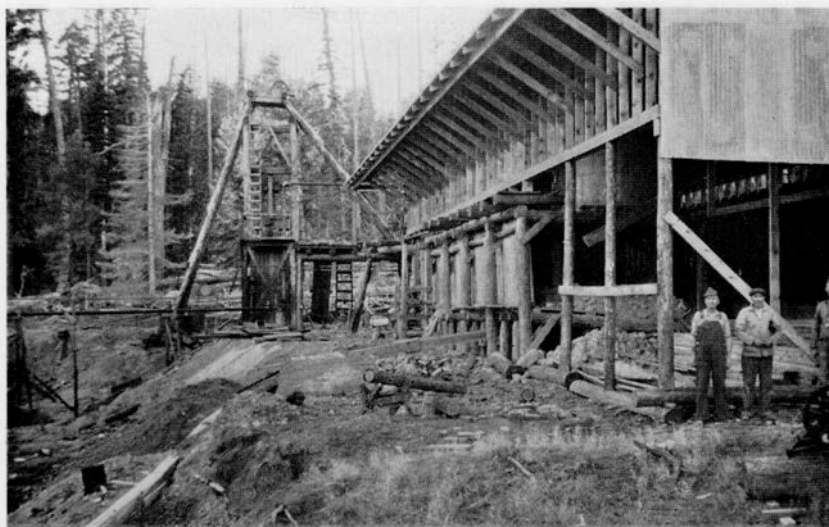
Photo No. 14—The shaft of the Blue Ridge Mine from which high grade ore was being hoisted for treatment in the retorts at the right. The man at the left is W. J. Westerling the discoverer of the mine.
