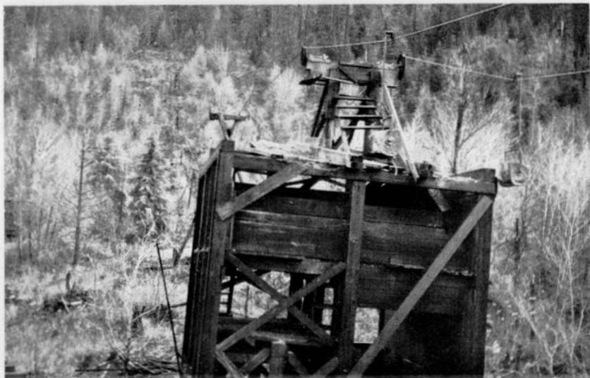
Photo No. 31—Black Butte Mine. Aerial tram which brings ore down from No. 9.
