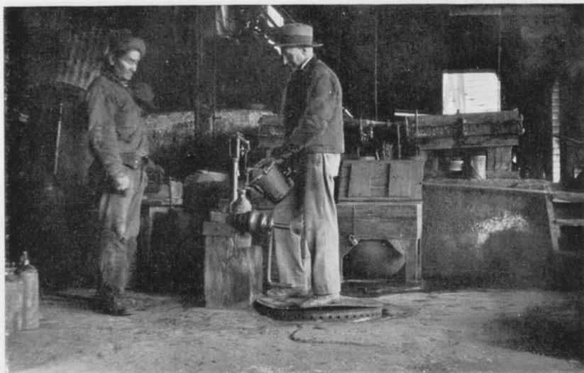
Photo No. 6—Filling the flask. Note the double soot pans in the background. Steam enters the lower pan to heat the upper one.
